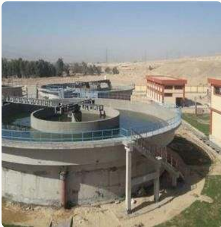
Clarifiers at a treatment plant
