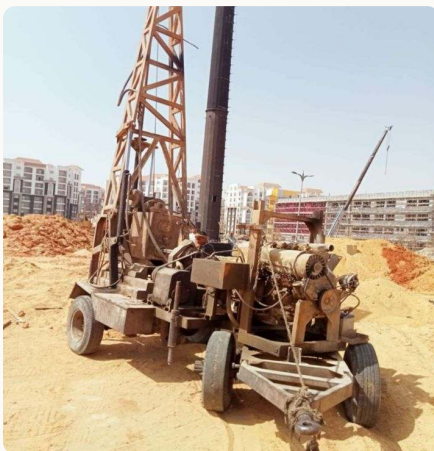
Borehole drilling on site
