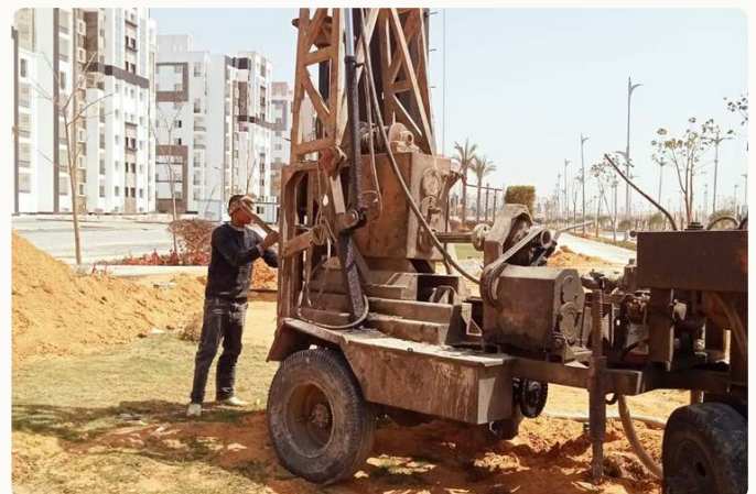
Crawler-mounted boring rig
