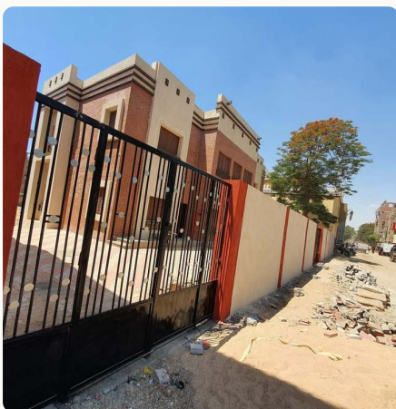
Boundary wall and entrance
