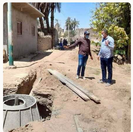
Manhole construction
