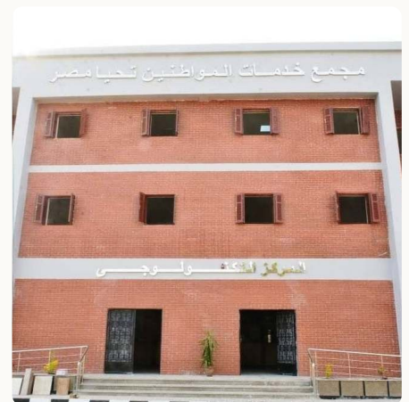
Services building — El-Ahaywa Gharb, Akhmim
