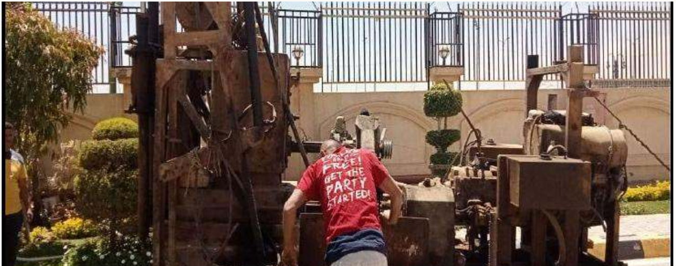
Field soil boring and site investigation works — Sohag
