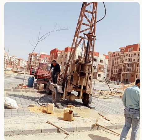
Boring crew at work
