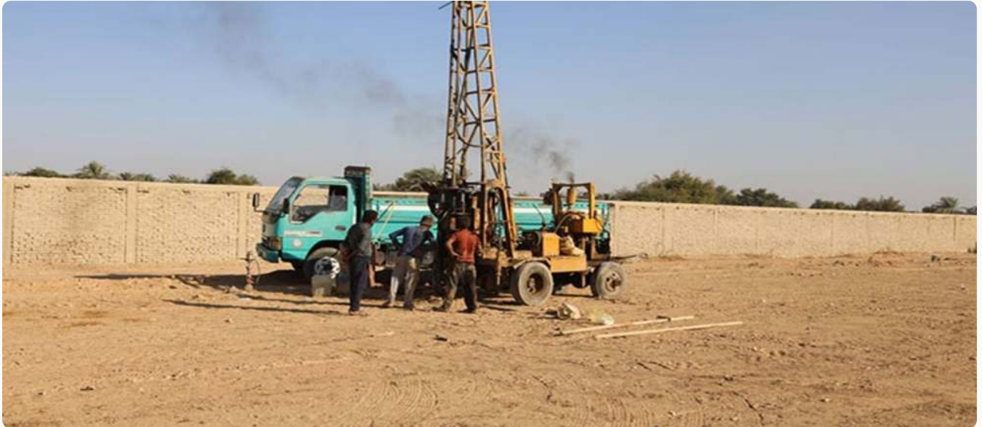
Boring rig on a project site
