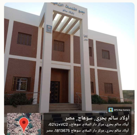
Services building — Awlad Salem, Dar El-Salam
