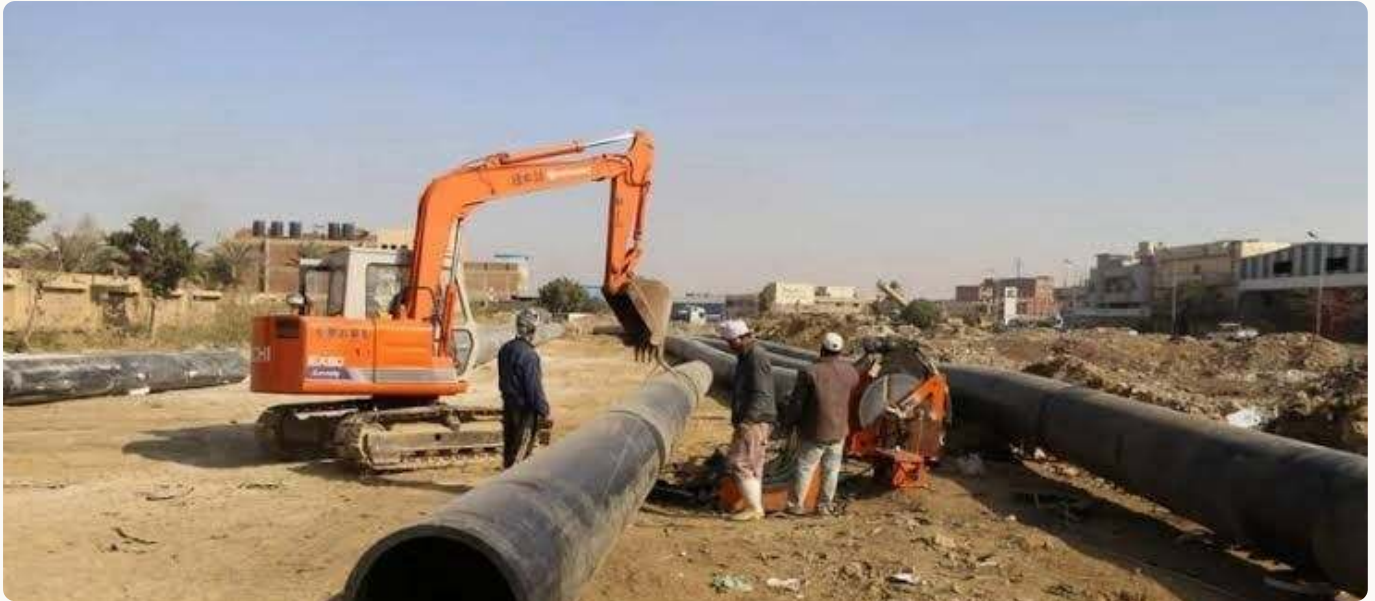
Laying main pipelines
