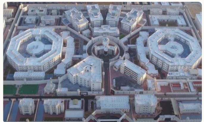
Aerial view of the buildings
