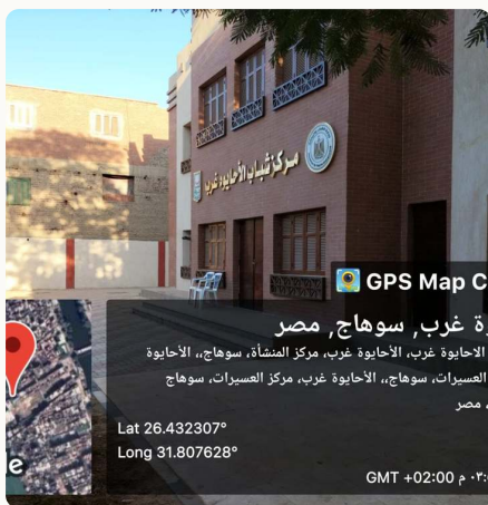
Services building — El-Ahaywa Gharb
