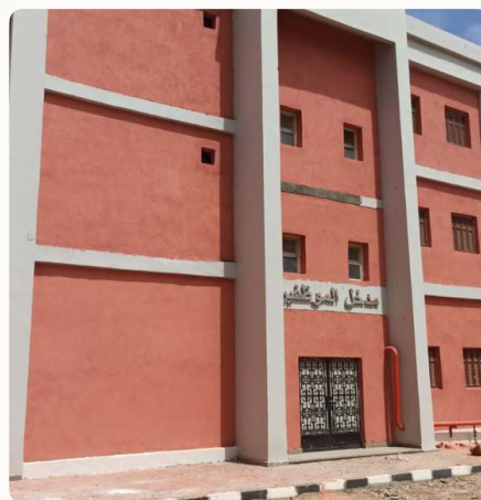
Services building — Tama
